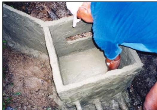
By now the second layer of mortar should have set. Mix a small batch of mortar (1:3 cement:sand) with waterproofing compound. Plaster a thin (3mm) finishing layer over the entire tank. Let the box cure overnight.
