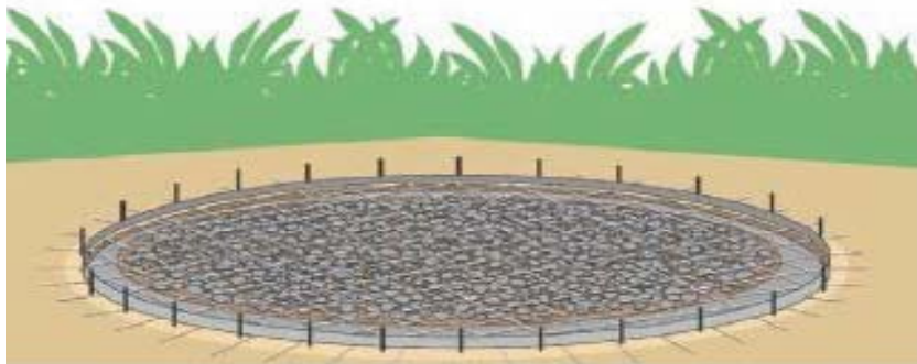
b. Plain GI strips and rebar ring comprise the base mold; a base course of gravel is laid.
